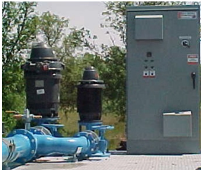
Outdoor NEMA 3R multiplex pump solution
